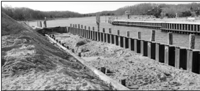
Bulkhead replacement construction
