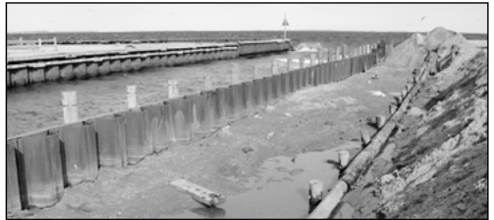
Bulkhead replacement construction
