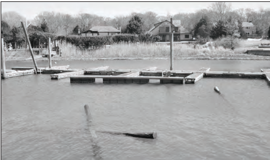
Damage to the marina poles on the floating dock
