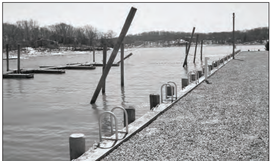
Marina pole damage by the bulkhead.
